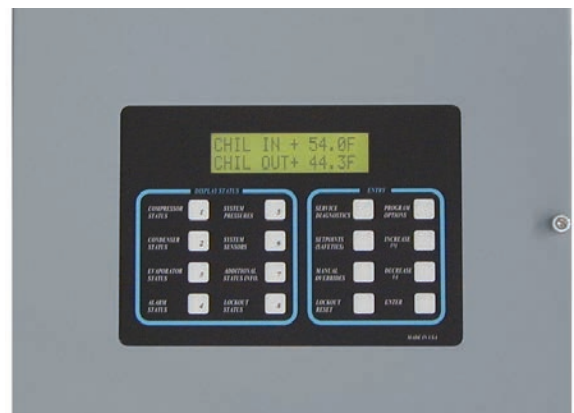
New MCS-8 Keypad mounted on door enclosure
